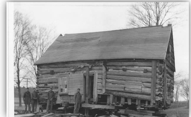
The Hyde Log Cabin during a 1941 restoration, when it was moved to its present location. Source: Grand Isle Historical Society
