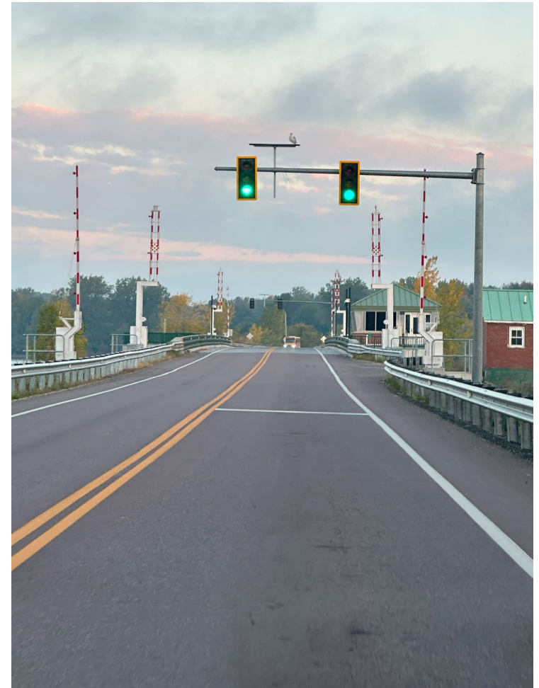
Grand Isle Draw Bridge on Route 2
