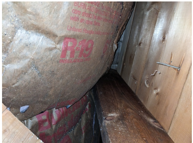
Attic has R-19 Fiberglass Batt's on the Ceiling
