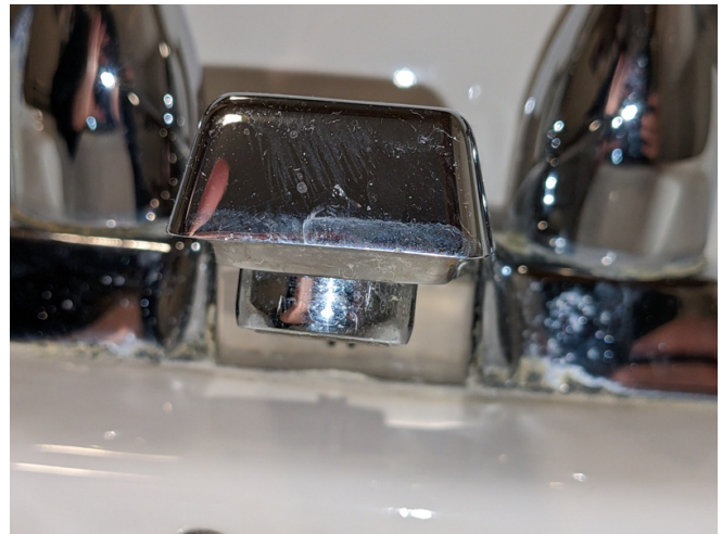
2.2 GPM Rated Restroom Faucet
