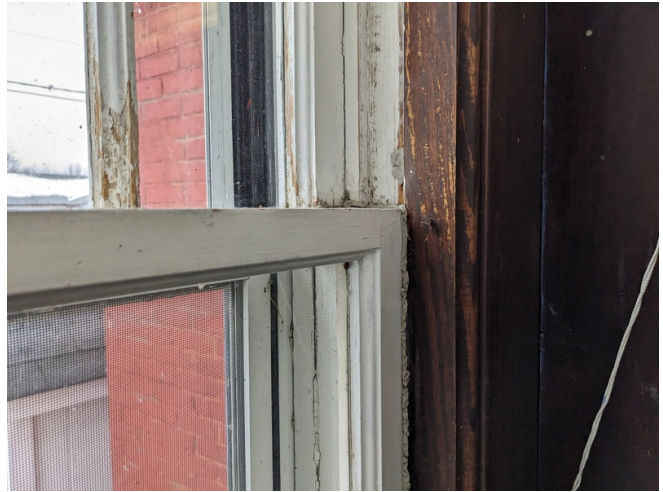
Window Sealed with Putty
