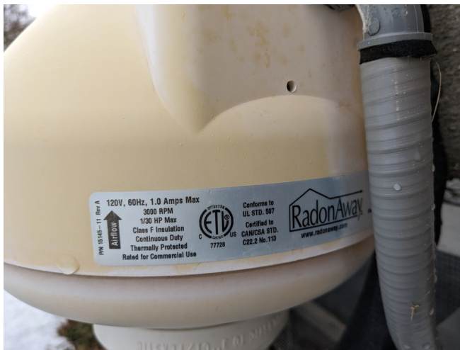
Basement Exhaust Fan by Radon Away
