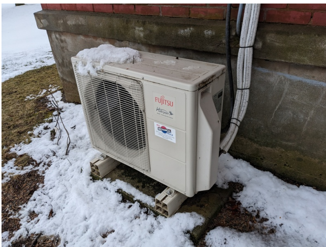
ASHP Condenser by Fujitsu
