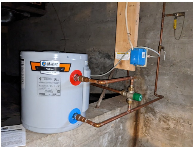
DHW Tank in the Basement
