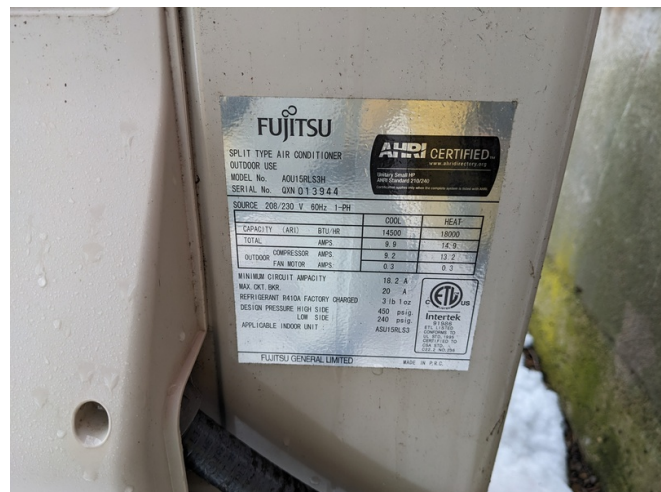
ASHP Condenser by Fujitsu; Model AOU15RLS3H
