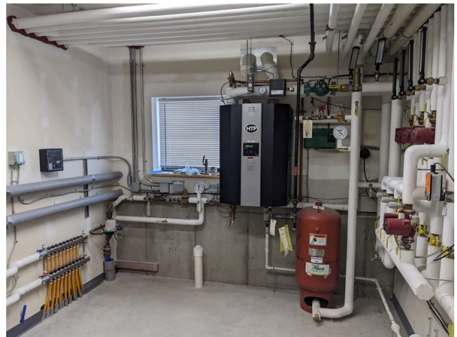
Mechanical Room Boiler and Hydronic Distribution
