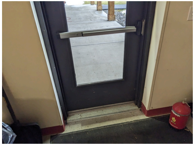
Drafty Entry Door; South Wall of the West Garage
