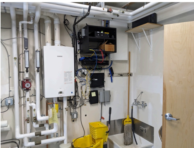
DHW Boiler in the Mechanical Room
