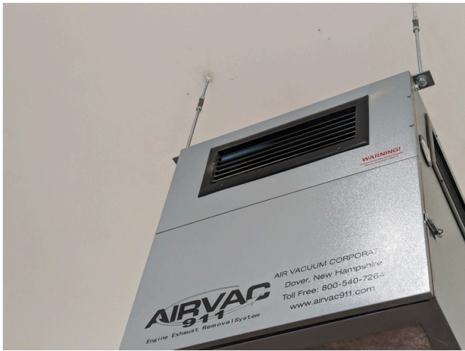
Vehicle Exhaust Air Filter by Air Vac
