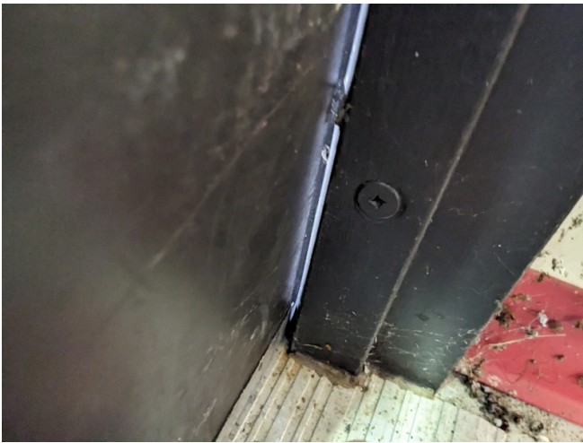
Draft Around West Garage South Entry Door
